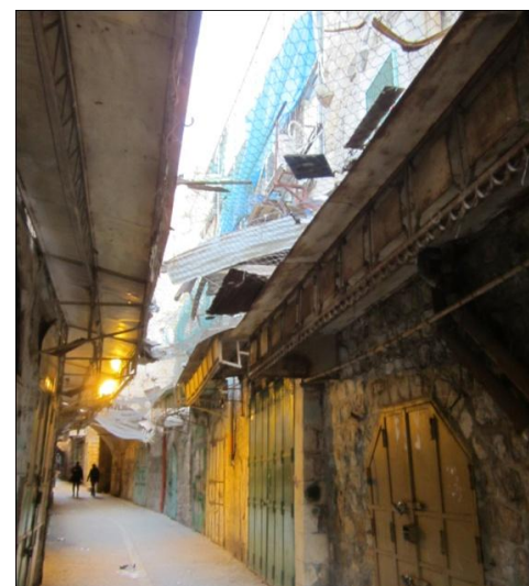
The souq in Hebron. There is a chain-link barrier covering the walkway because the Israeli settlers that live above the market regularly throw waste, eggs, and other debris from the windows to discourage business in the souq.
